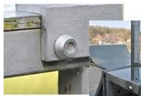
Armour Ring Installed
